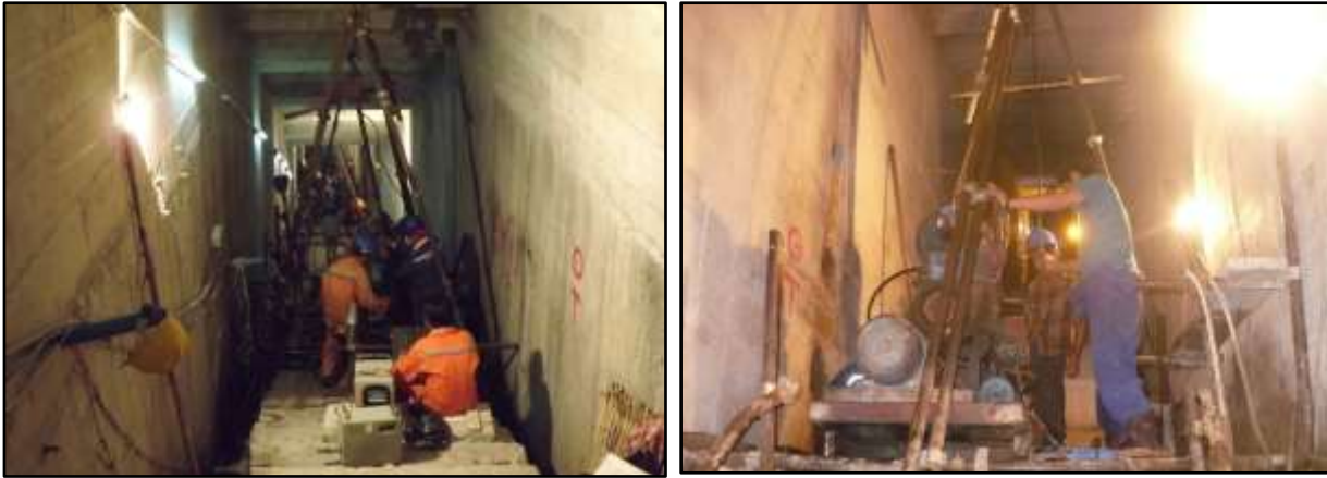
Figure (16) Curtain grouting inside the foundation gallery at UPL dam
